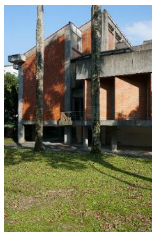
Recent photo of the Former Academia Sinica Center for American Studies building. © Yao-Ting Wu
